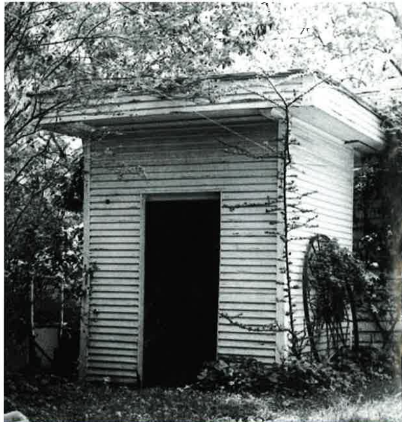
During Dr. Payne's ownership, a generator and batteries in this small outbuilding provided electrical power for Winterham's lights. Courtesy of the Ruth E. Lloyd Information Center (RELIC).
