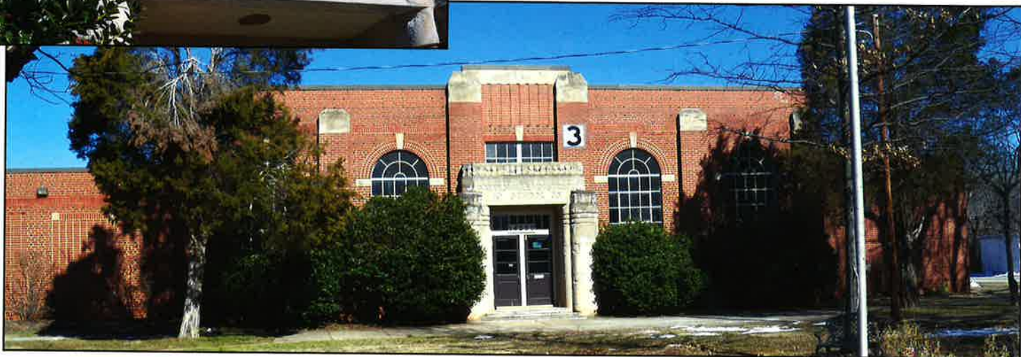
Located on Rt. 55 east of Haymarket, Gainesville Elementary School was opened in 1935, and expanded several times. It now serves as the PACE West School. Inset: Entablature above the front entrance to the old Gainesville Elementary School includes the date of its opening, 1935.
