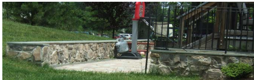
Stone Retaining Wall
