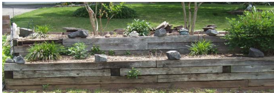
Wood Retaining Wall
