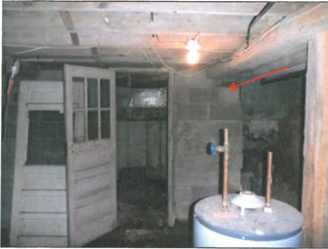
Photo 4 – View of foundation showing some settlement and dirt crawl space Photo 5– View of foundation showing settlement crack at corner.
