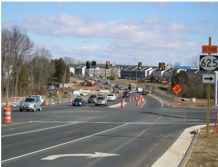
Intersection of Heathcote Boulevard and Route 15
